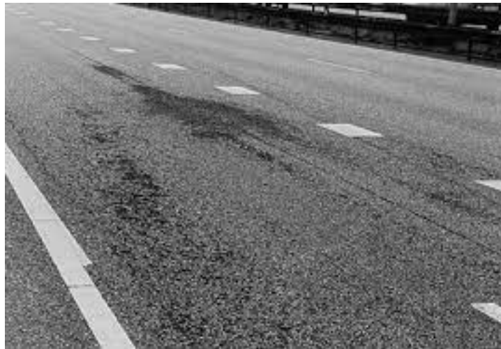
Figure 1: Ravelling of PA in the Netherlands [12]
