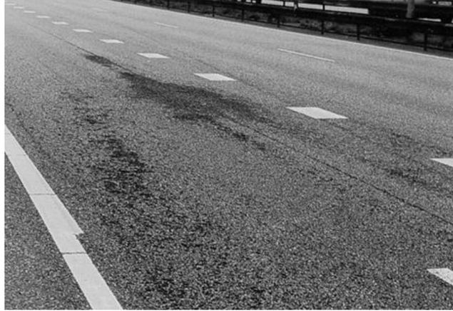
**Figure 2.2:** Ravelling of porous asphalt in the Netherlands. Adapted from [1].
