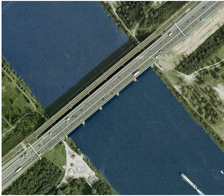
Figure 1: Picture of the bridge "De Hollandse Brug", which connects the province Flevoland to the province North-Holland in The Netherlands.
